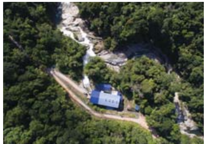
Amcorp Perting Hydro 6MW, Bentong, Pahang.
